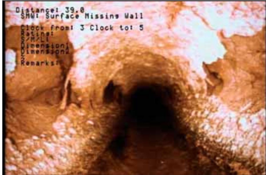
A section of the 1947 pipe, showing the complete erosion of the sidewalls.
